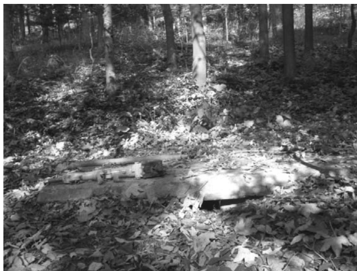
Fig. 3. Research Position No. 3. The well covered with a concrete slab – emissions from inside the well; the commune of Iwonicz-Zdrój, Subcarpathian voivodeship, 2011 (photo by Lipińska E. J.)
